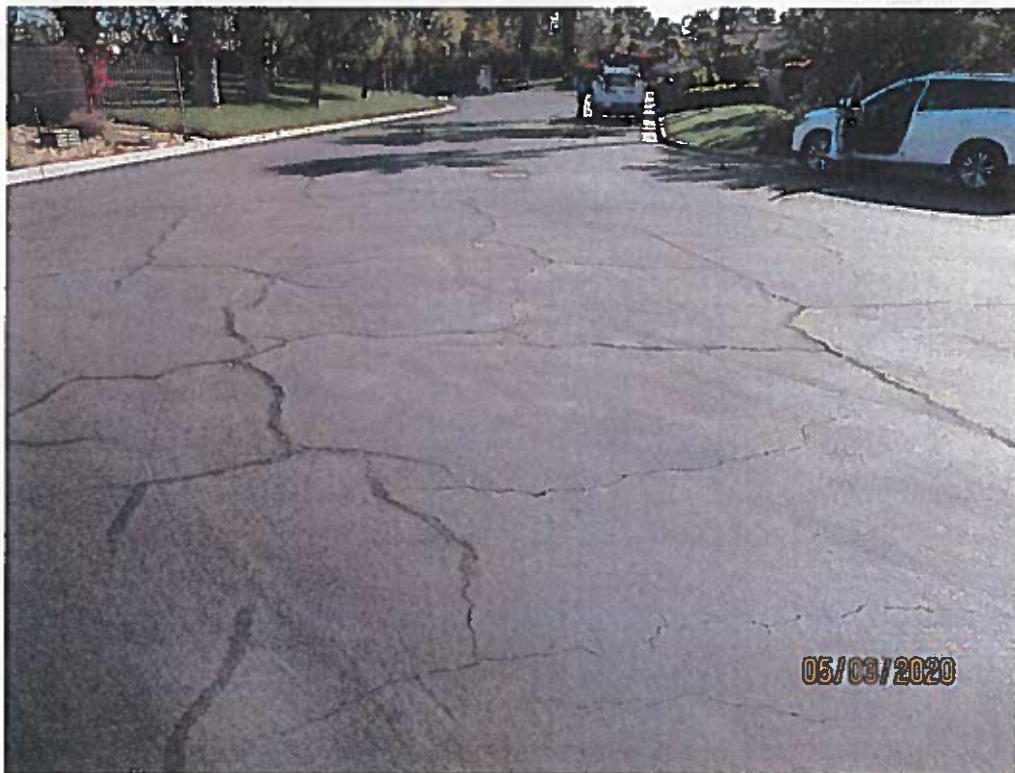
PHOTO 8 Continuous slight to severe block cracking is depicted in this photo.
